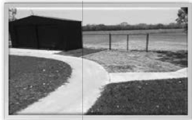
LA Establishment Grant Manyallauk Crèche Project – Roper Gulf Regional Council – 2014
