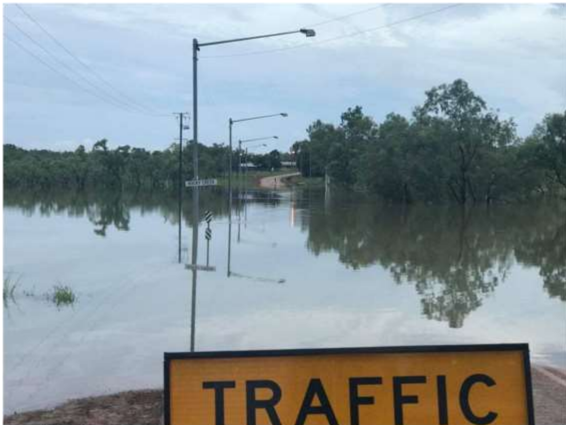
Australia Day 2018 – Flooding
