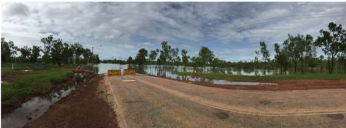
Australia Day 2018 – Flooding
