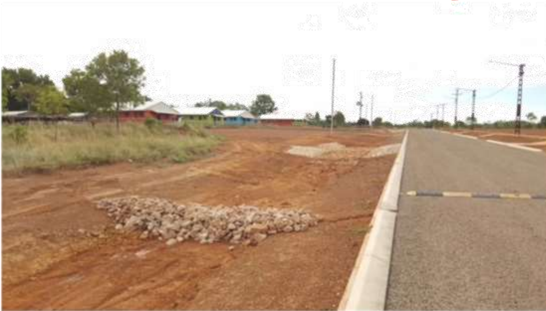
03 – Rock check dam reinstated. Drain scouring fixed.
