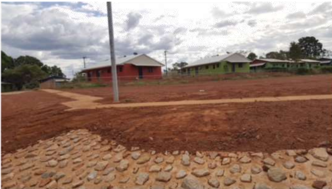
08 – Scouring above culvert 1 fixed. Footpath cleaned
