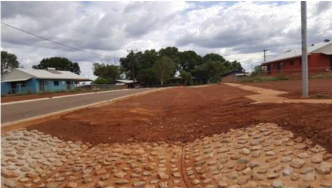
09 – Protection works above culvert 1 cleaned. Scouring fixed.
