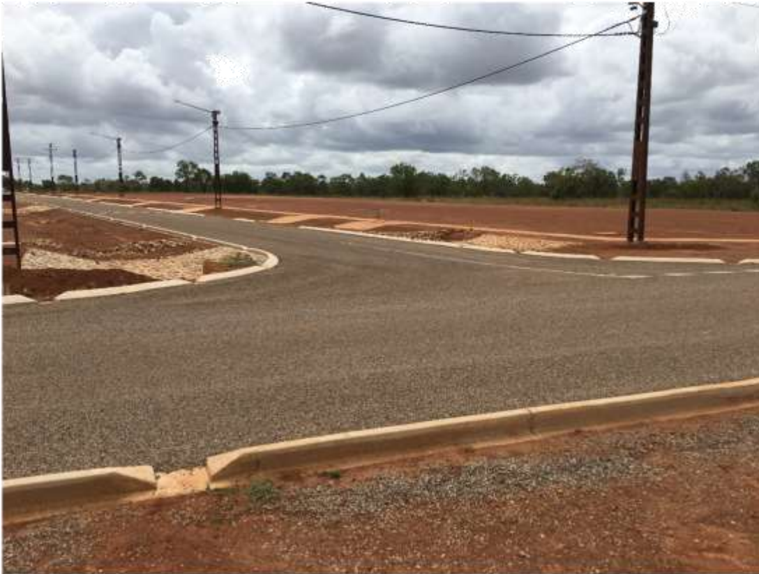
15 – Roads are clean with no defects identified
