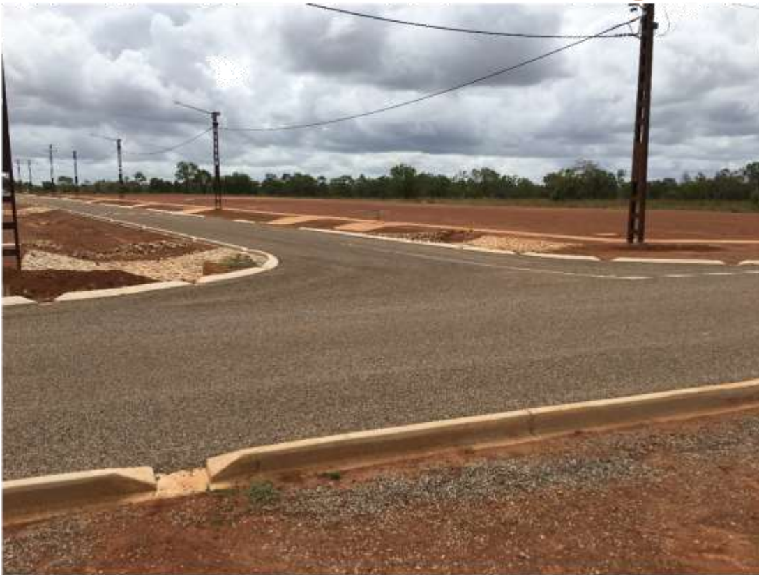
15 – Roads are clean with no defects identified
