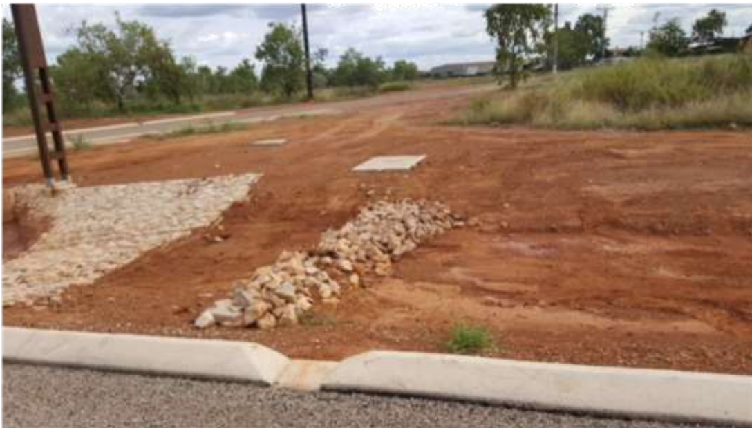
02- Rock check dam above culvert 4
