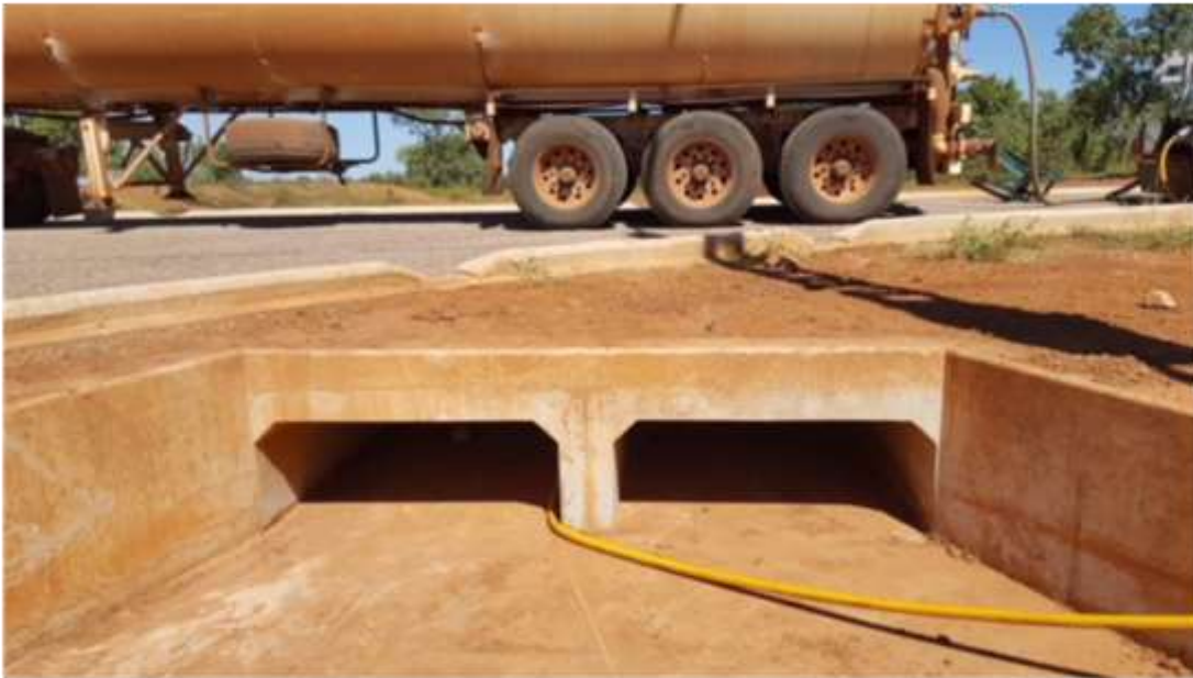
11 – Culvert 4 cleaned out
