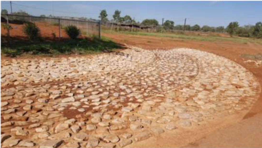
21 – Stone pitching drain protection at the bottom of Rainbow Street has been cleaned
