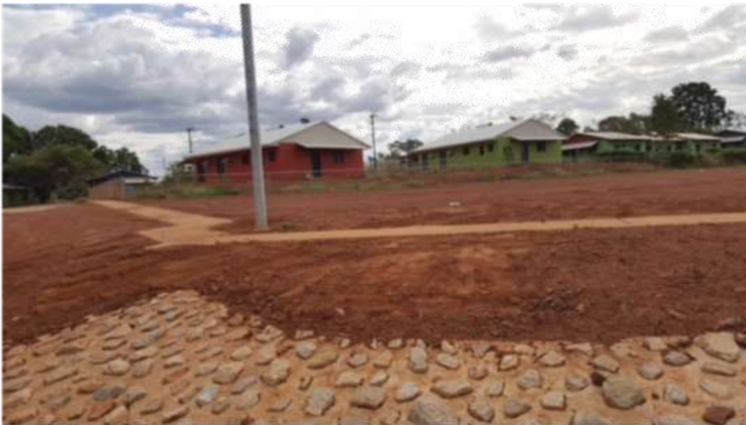
08 – Scouring above culvert 1 fixed. Footpath cleaned
