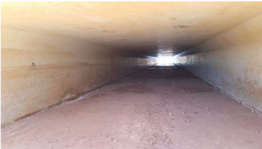
12 – Culvert 4 cleaned out
