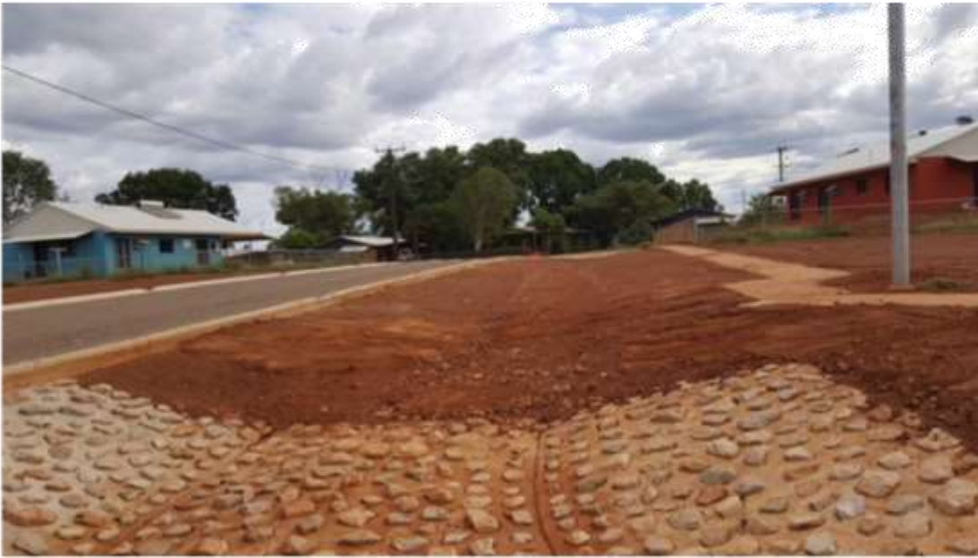
09 – Protection works above culvert 1 cleaned. Scouring fixed.
