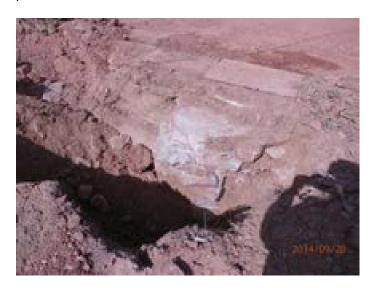
The restriction in flow caused by this pit arrangement is causing the silt and dirt to settle out and block this full length of pipe. This fault was built into the original system and the stormwater system in this area is not likely to have been functioning for a number of years.
